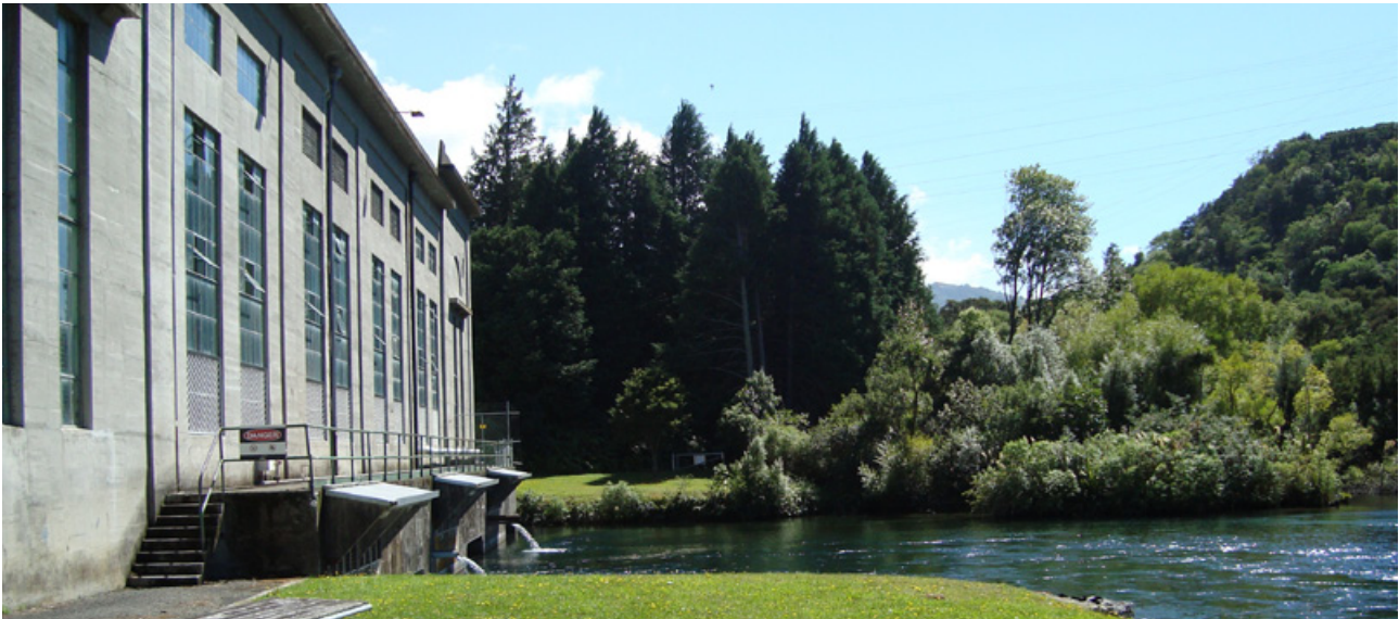
The generator hall and the tailrace into Lake Whakamarino. Ergo Consulting was involved in the design of the control system replacement at Tuai Power Station, from which water passes through and is discharged into the lake. Image courtesy of Ergo Consulting Ltd.
